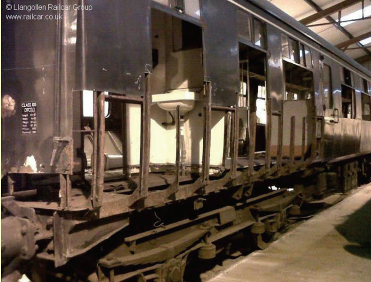
Progress maintained: with the front and middle saloon framework repairs and replacement panels now completed, the rear (and final) passenger saloon, including toilet area, has been stripped of its rotten metalwork ready for repairs, 10/12/12 (Llangollen Railcar Group)
